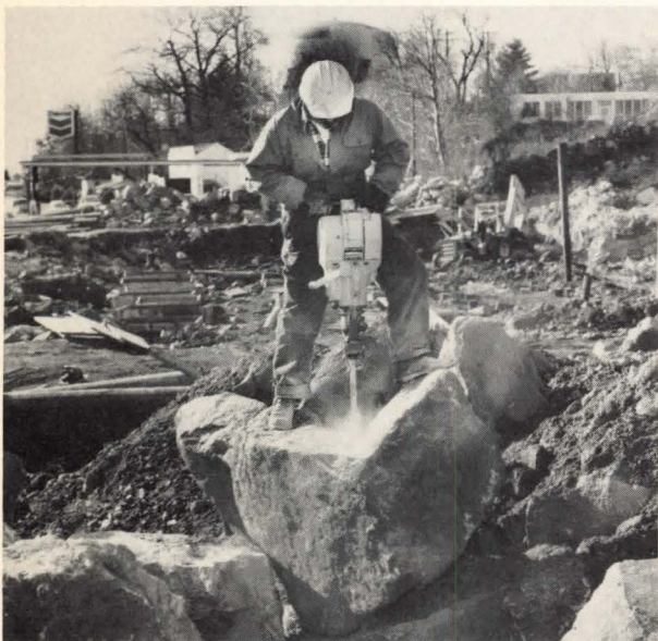
Gasoline-powered "Pionjar" (above) operates in a drill or impact mode. Versatile tool, which drills to a depth of approximately 20 ft., delivers compressed air to blow out the particles. Abema. Circle 247 on reader service card
