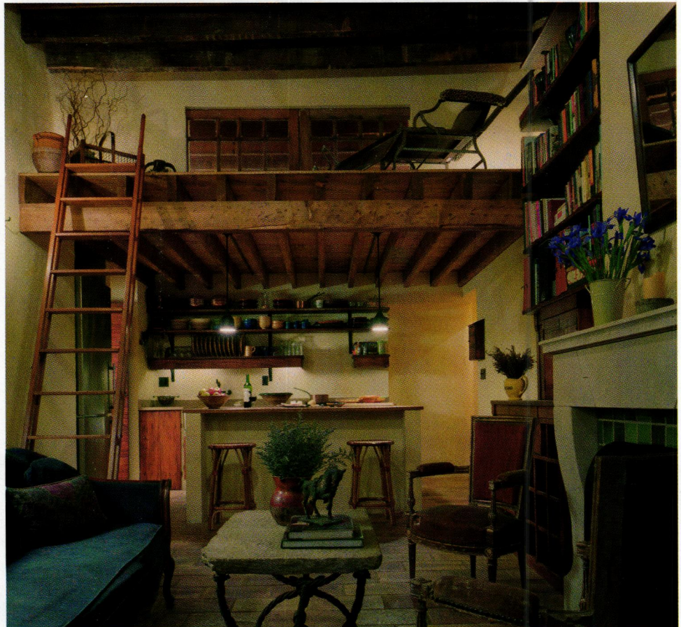
Salvaged beams were used over the kitchen to create a loft space. The team also incorporated salvaged windows into the space.
