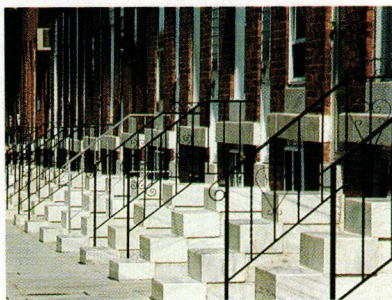
Marble quarried north of the city was used to build the steps that front many of Baltimore’s ubiquitous row houses.
