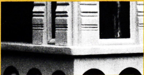
...sanded, nailed, stained or painted.
