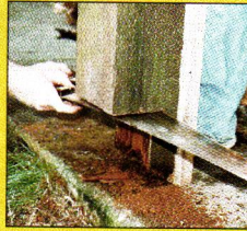
Rotted & infested base of a loadbearing column is completely sawed off and replaced with WoodEpoX .
