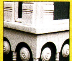
Consolidation and rebuilding of rotten windowsill with LiquidWood and WoodEpox .
