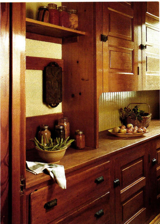
Stripped of many layers of paint, the existing pantry provided design cues for the new kitchen: cabinet depth and height, hardware, backs of beaded board.
