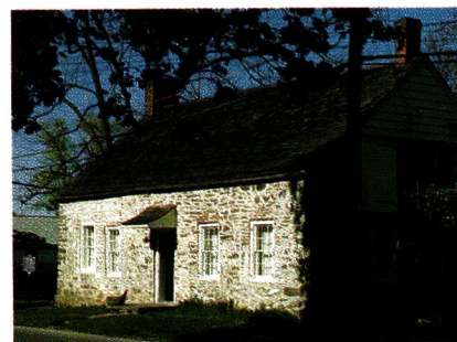
One of dozens of Huguenot stone houses extant in the Hudson Valley.
