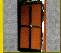
Antique window sash is salvaged, consolidated with LiquidWood and rebuilt with WoodEpoxy .
