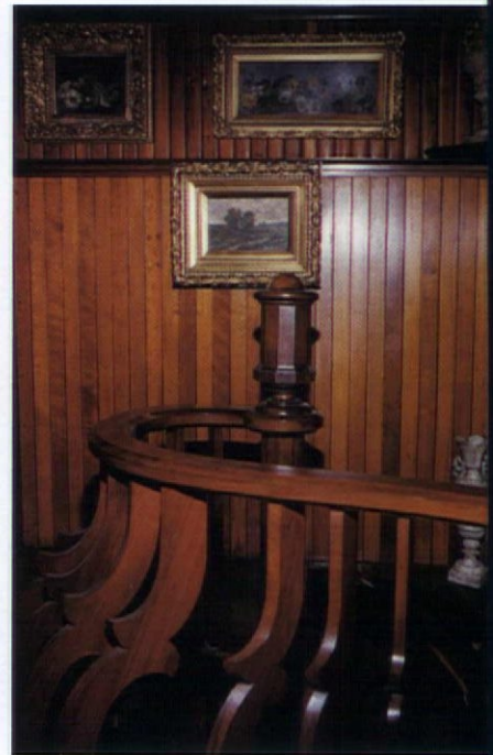
LEFT: The master bedroom is very Alpine: horizontal wood board walls, bare walls and floor. Unsigned furniture is reminiscent of Belter. The crazy quilt is one of the family's treasures. BELOW: The upstairs balusters are sawn walnut in whimsical patterns designed by Tinker.
