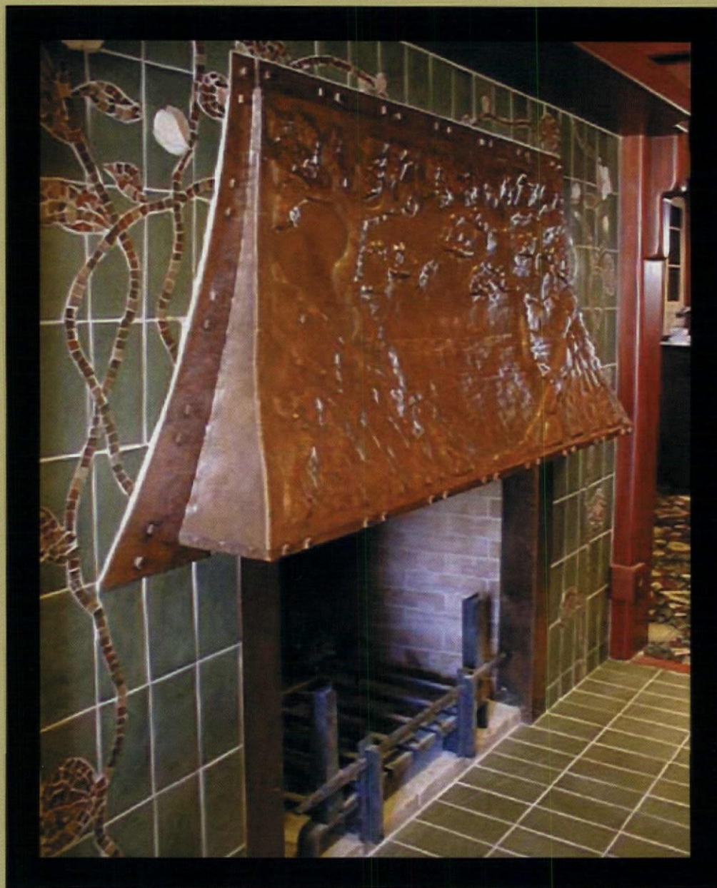
Hammered copper hood & wrought iron fire grate, The Lodge At Torrey Pines, La Jolla, CA
