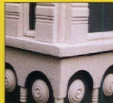
Consolidation and rebuilding of rotten windowsill with LiquidWood and WoodEpoxy .
