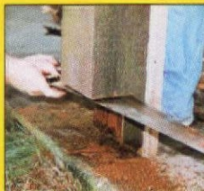
Rotted & infested base of a loadbearing column is completely sawed off and replaced with WoodEpoxy .
