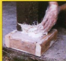
Rotted & infested base of a loadbearing column is completely sawed off and replaced with WoodEpoxy .
