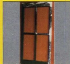
Antique window sash is salvaged, consolidated with LiquidWood and rebuilt with WoodEpoxy .
