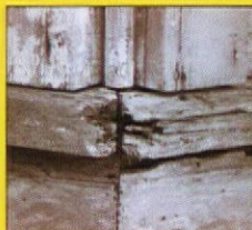
Consolidation and rebuilding of rotten windowsill with LiquidWood and WoodEpoxy .
