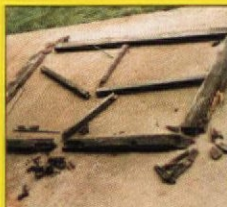
Antique window sash is salvaged, consolidated with LiquidWood and rebuilt with WoodEpoxy .
