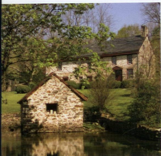
ABOVE: The spring house and main house at Kockert's Tavern. TOP: (left to right) Revival interior of a 1937 house in the farmhouse vernacular by G. Edwin Brumbaugh. A Georgian chimneybreast of 1739. Arts and Crafts-era English-style chimney in concrete and plaster. An early-18th-century staircase incorporated into an addition.
