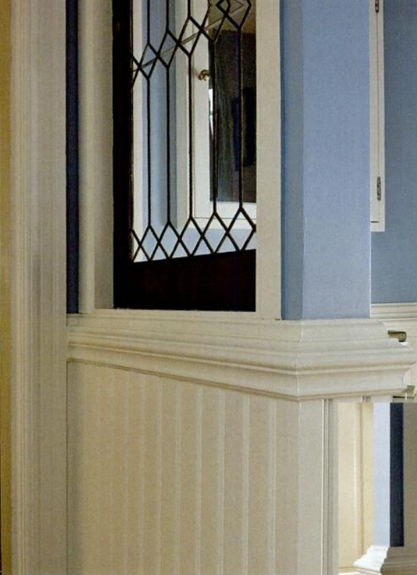
LEFT & BELOW: Carpenter Jeff Loux created a short wall divider out of beadboard and a salvaged leaded glass window, enhancing the sense of privacy between bedroom and bath. The waterfall sink, patented in 1911 is a salvage piece. Water flows out beneath the porcelain bump at the center of the basin. BOTTOM: The under-the-stairs powder room is lusciously Victorian. Its original door (which opened into the dining room) was relocated to the hall. In its place is a stained glass window that adds to the jewel-box effect.
