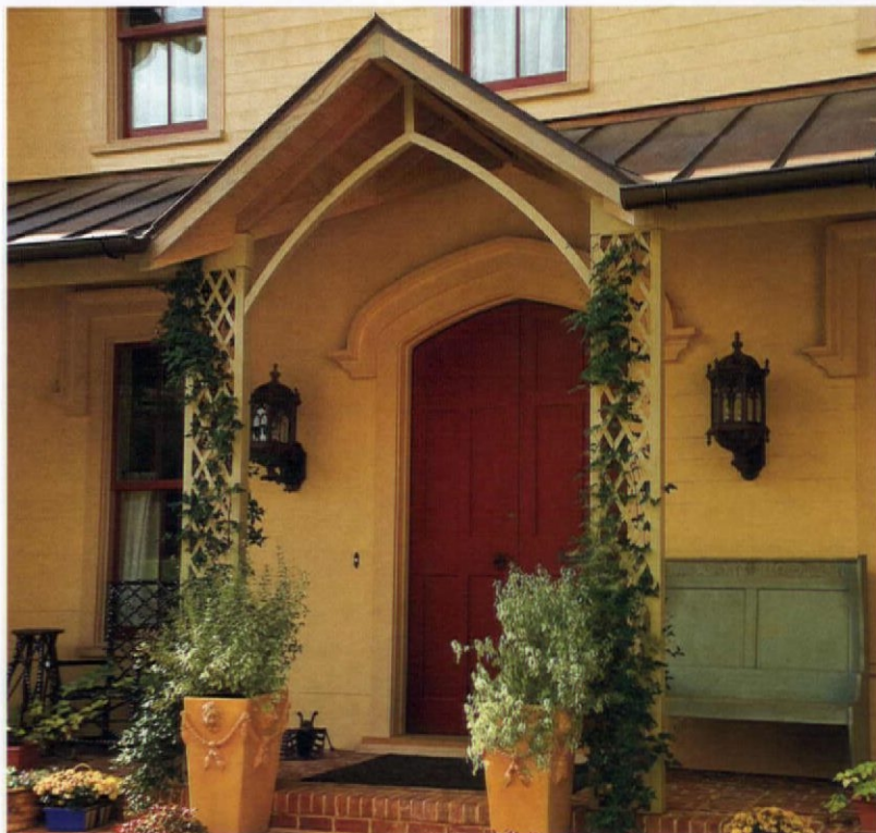
BELOW: The understated country entrance has lattice posts and a simple spanning arch made of steel. The owners found a pair of 250-year old Gothic doors with original hardware from a cathedral in England, which had been exported to Lynchburg, Virginia. The heavy lanterns were found on eBay. Antique stick furniture is from the Catskills.
