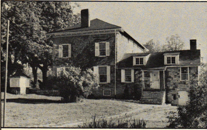
The 1696 Dutch Cottage is attached to rear of main house. The back wall collapsed in 1924. Stephen reconstructed the wall, using stones from the property, following the original foundation line. He also built the window sash in the re-created wall, using the neighboring window as a pattern. The workshop where Stephen creates reproduction light fixtures is in the cellar of the Dutch Cottage section.
