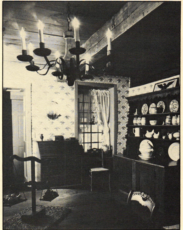
In dining room in the Dutch Cottage, modern plaster ceiling was removed to expose smooth hand-hewn beams and attic flooring. Light fixture is Stephen's handiwork.
