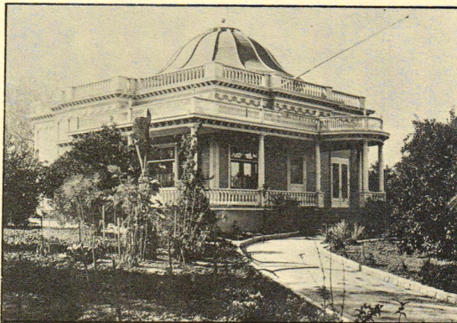
This is the way the manor looked before the decorative dome was removed. The Wilmots hope to have a fiberglass dome put back on and the railings restored for the Redlands Centennial in 1988.
