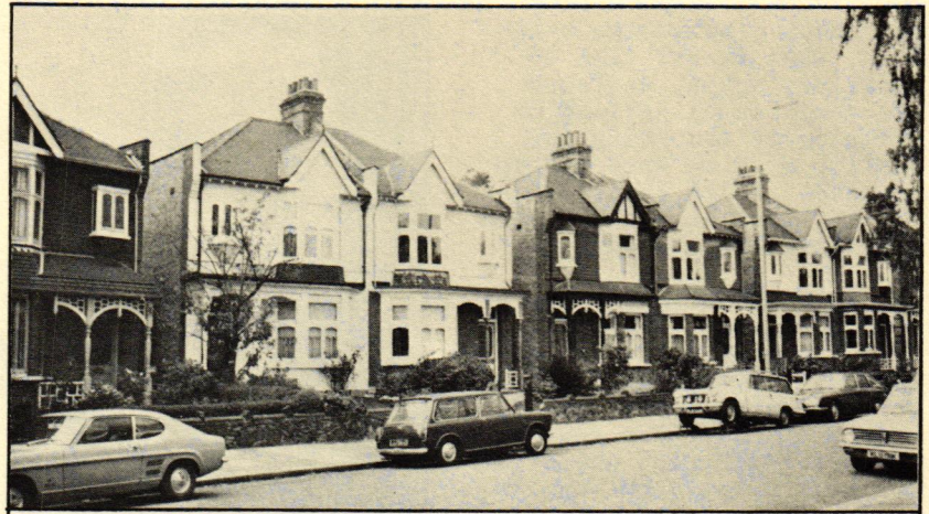
The Gadsby's house on Farrer Road, one of London's many streets of row houses. Note the number of chimney pots--very few older houses have central heating in England.
