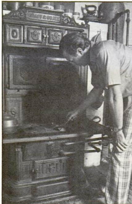
Don Yule pokes the fire in his kitchen stove. The water front is below the cooking surface where the two pipes carry water to and from the hot water tank on the side.
