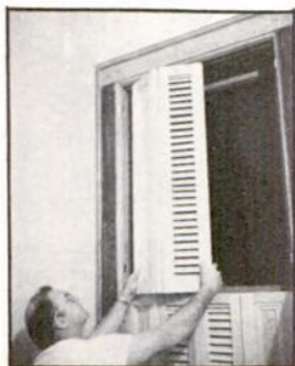
Paul Griffith fits shutters to out-of-square window.
