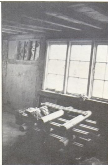
The leaded glass window, exposed after 200 years, is in the corner. Stacked in front are solid oak mullions and ceiling bosses.
