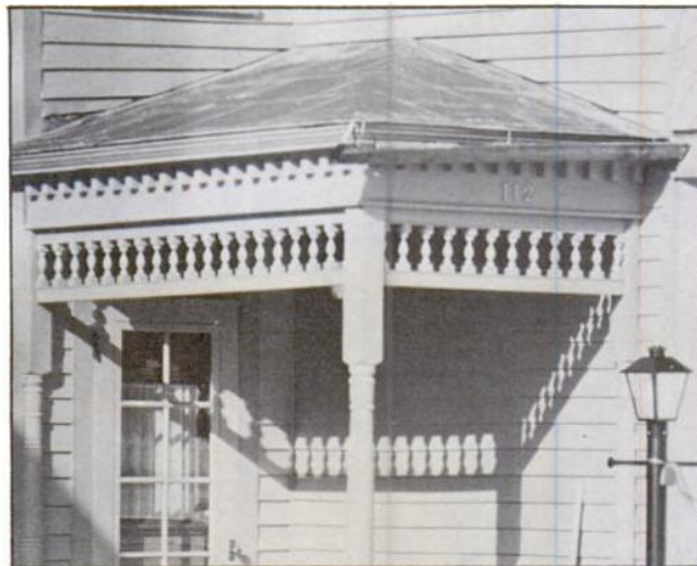
Porch after restoration was completed.
