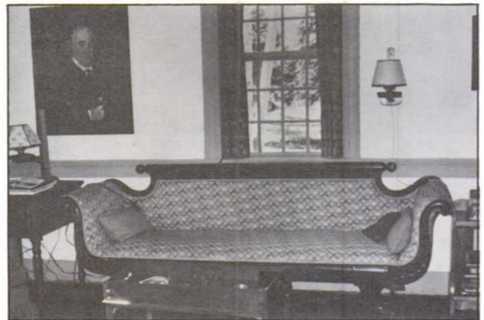
The glass pieces installed for insulation do not detract from the appearance of the twelve-over-twelve windows.
