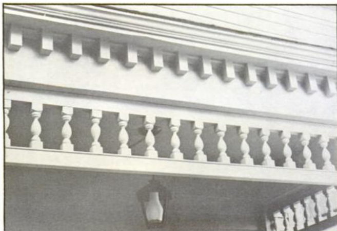
Detail of spindles used to restore porch.
