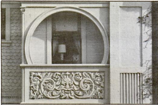
The top sash of the window seen through the arch has small panes as a border. Other details frequently found in the Queen Anne style: Decorative panel, dentils, columns, varied texture of brick, board and shingles.
