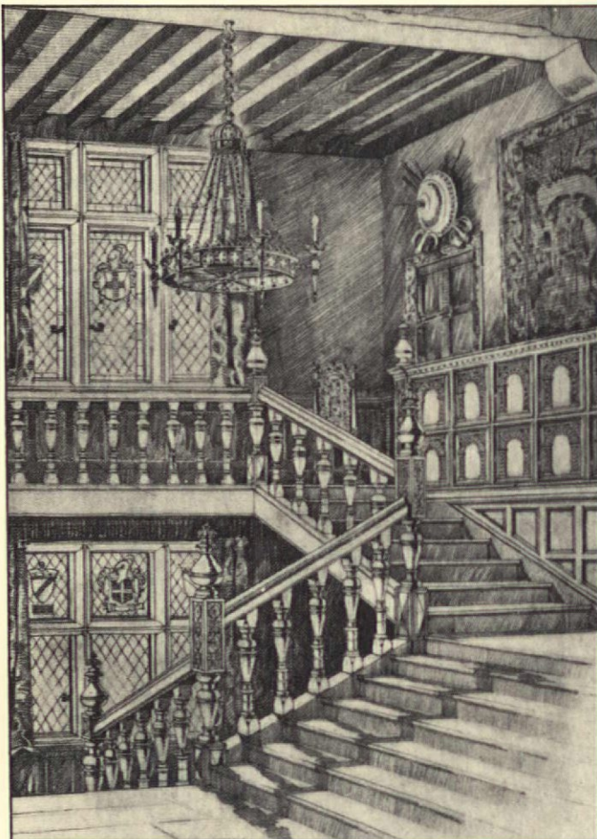
The main staircase from Sheldon Hall, in Leicestershire, England. It was characteristic of the first wooden staircases to build them around a square well and break them up into short flights with a low pitch.
