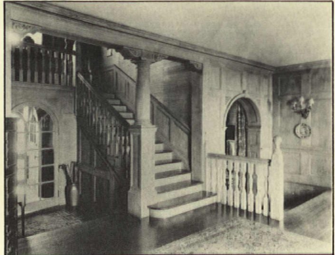
This is the entranceway of a Tudor style house, built in 1914, in Waterford, Conn. Typical of Tudor revivals, the walls are oak panelled and the floor is polished oak.
