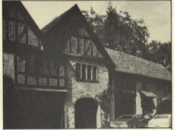
Not as commonly found in the American versions, this 1929 Pennsylvania Tudor has varying brick patterns in the "nogging" between the beams. These decorative brick patterns were often used in old English half-timbered houses.
