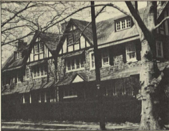
A typically American Tudor built c. 1914 in Pennsylvania adds Colonial features (shed dormer, shutters) as well as regional characteristics (fieldstone front, pent roof over the oriel window) to the old English form and half timbering.
