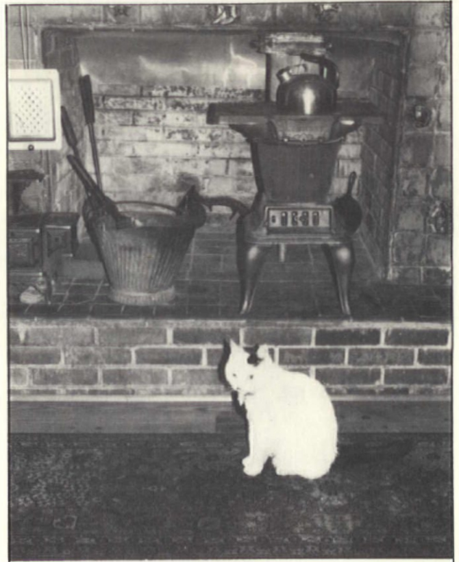
In this close-up photo of the fireplace and stove, you can see the piece of aluminum wedged in place behind the stove to direct warm air into the room.
