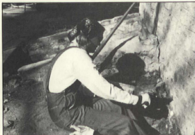
Norma did much of the preliminary work before professionals came on the job. Here she is drilling holes for the power lines through 18-20 in. of the fieldstone. It was a three hour job.
