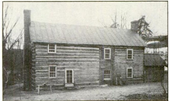
Back view showing the three original log houses, plus (at the right) the recent addition that houses the furnace, water-pump and hot-water heater.
