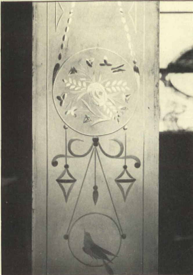
Cut glass panel from an inside entryway. The design areas are "brilliant" because they were polished after being incised by the cutting wheel. Although incorporating only "lines and spots," the artist was able to produce a wide variety of realistic figures.
