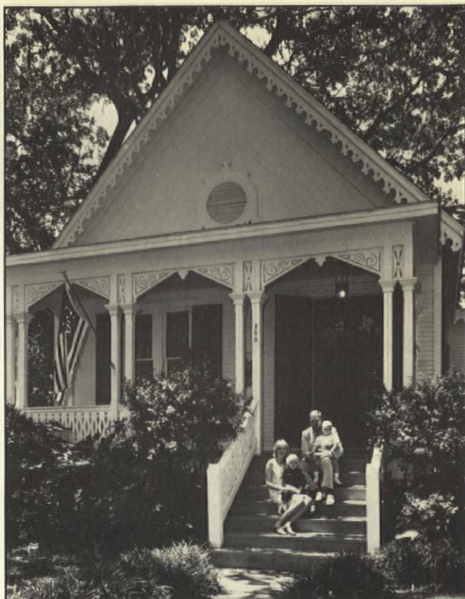
The Ray family, early members of the Council, live in this Steamboat Gothic home in Mobile's Oakleigh Garden District. Purchasing the house in 1971, the Rays have done extensive patching, painting, stripping and refinishing. One major project involved replacing floor furnaces with central heat and air conditioning.
