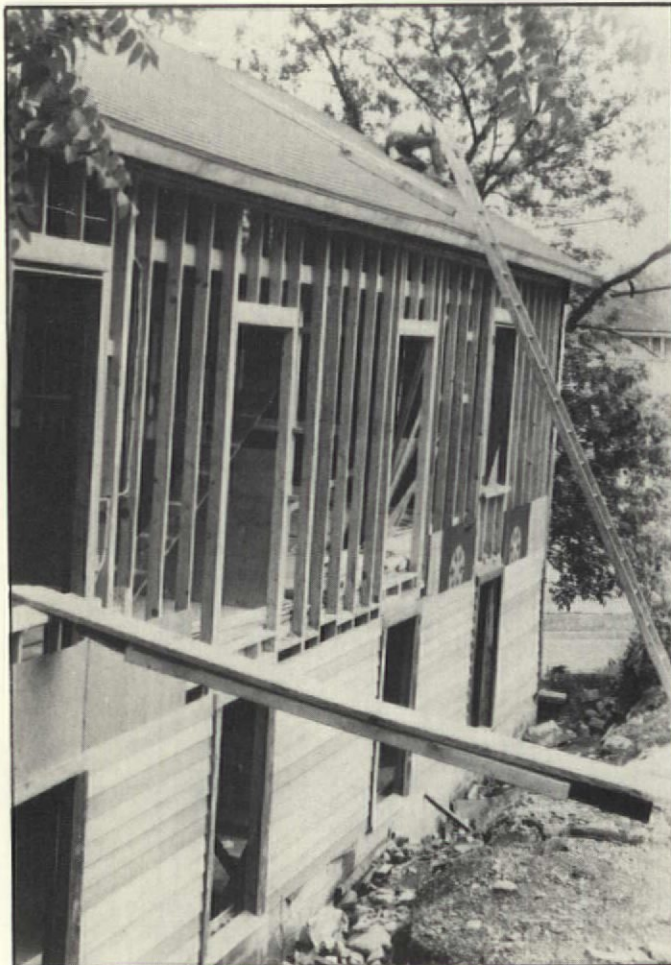
View of the east wall being reconstructed with the balloon framing.
