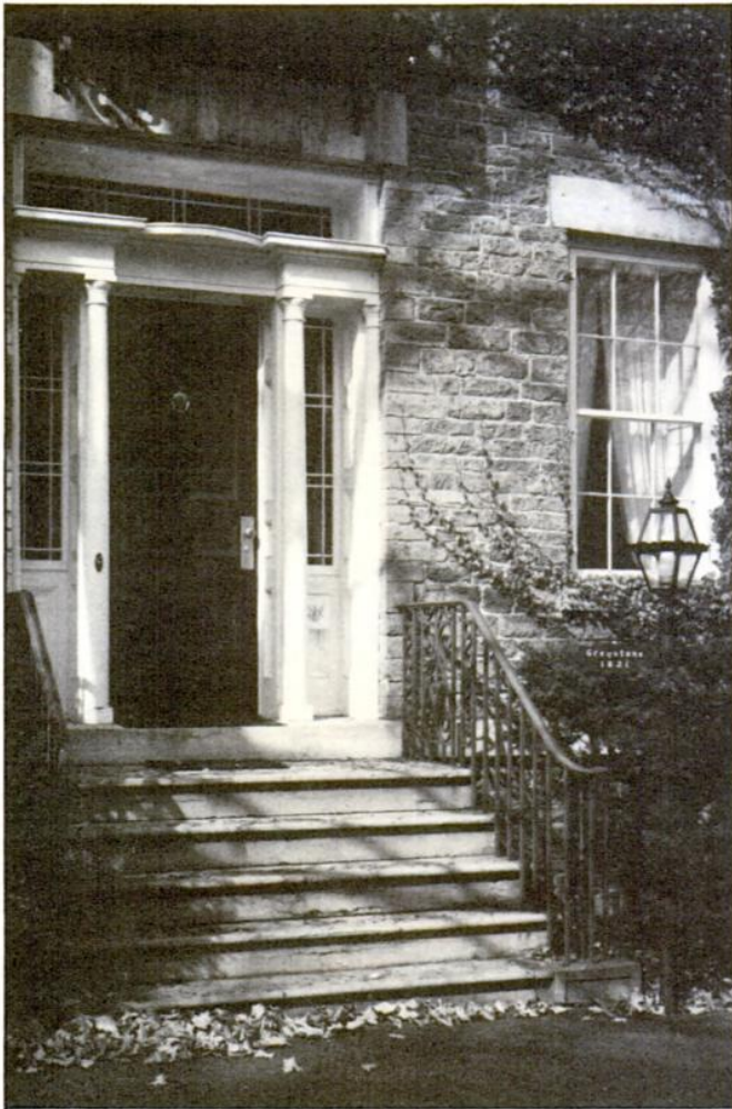
The main entrance is the only touch of richness on the classically simple facade. The paint was burned off the entranceway and it was painted white with a black trim.
