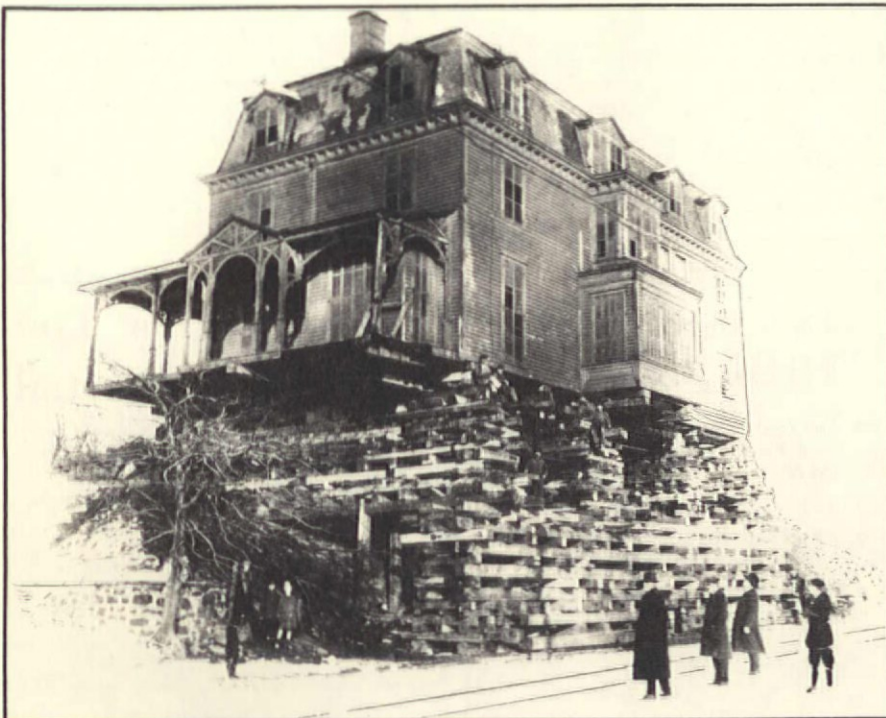
This remarkable move took place in Brooklyn in 1923. The Perry Mansion was moved across the street and to lower ground. Because traffic could not be interrupted, a sophisticated cribbing was built to extend over the roadway. The structure was pulled across and re-situated 200 feet from its original site.
