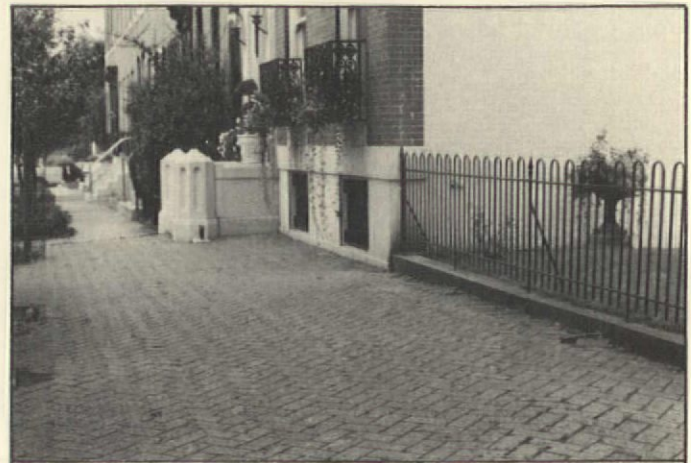
This herringbone walk has aged to a beautiful deep red patina in the century or more it has served in front of this house in Baltimore.
