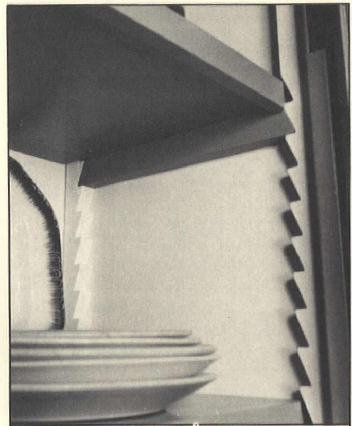
A traditional system for adjustable shelves.
