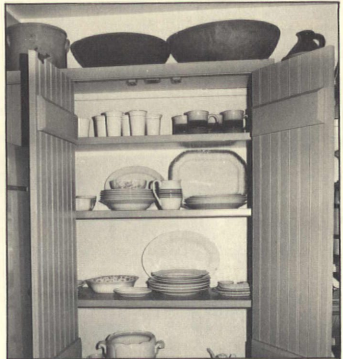
The larger cabinet: Notice the battened doors and the appropriately thick shelves.
