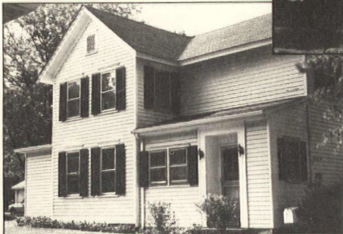
The Sachs' house in Cranbury, N.J. The door was probably on the front facade at one time, but previous owners moved it around to the side when they enclosed a porch. The Sachs will leave it as it is, because the air lock prevents wind from whizzing into the house.
