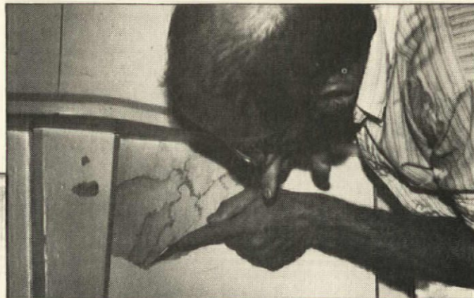
The mantel was originally marbled. Chemicals would remove marbling as well as paint, so a scalpel will be used.
