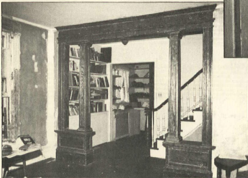
The partially-stripped chestnut woodwork, between parlor and enclosed porch
