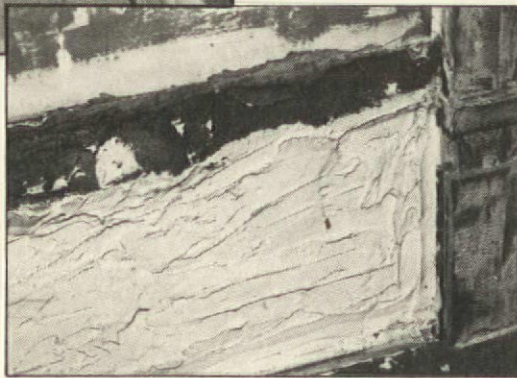
The circular mark hints at a lab cork plugging a hole made by the insulation contractor. It will be invisible after a good paint job.
