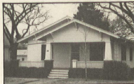
THE ORIGINAL: This Craftsman Bungalow retains most of its original detailing: knee braces at the eaves, elephantine columns on the front porch, narrow clapboard siding, and a delicate porch balustrade that forms a vertical counterpoint to the horizontal siding.
