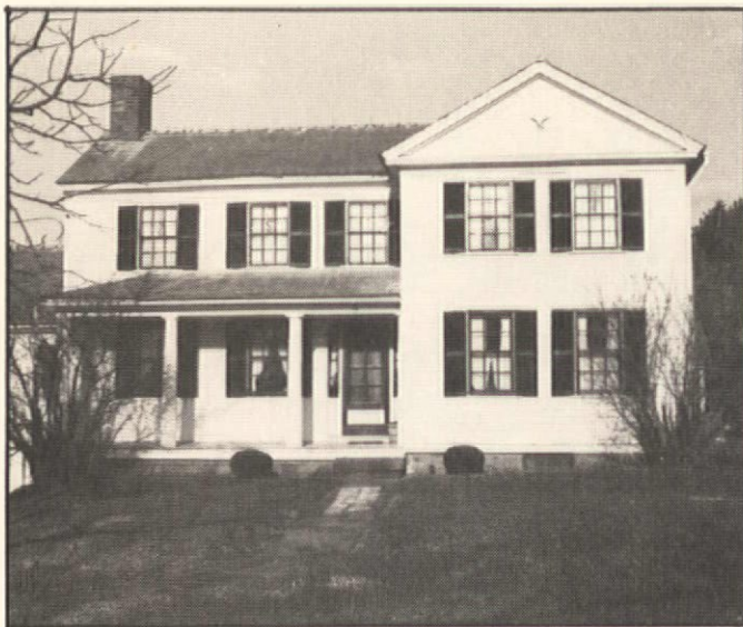
The Greek Revival house, with its emphasis on the prominent gable, was the direct ancestor of the Homestead House. This 1820 farmhouse has mouldings attached to the main gable to suggest the pediment of a Greek temple. Stripped of its Greek detailing, this same type of house was being built a century later in city and suburb. Then, they called it simply a "modern house." We are calling it the Tri-Gabled Ell.
