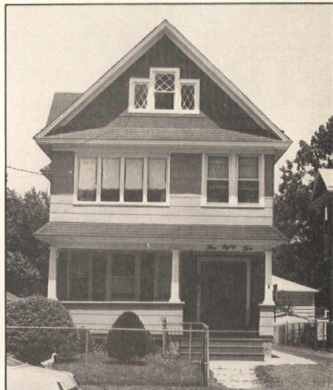
This 1920's Homestead House is typical of thousands built in city and suburb in the early 20th century. Though partially remuddled, its relationship to the 1820's Temple House is clear. The biggest difference is the porch that extends across the front facade. Note also the triple window in the gable. Its shape suggests a Colonial Revival Palladian window, while the diamond-shaped glazing evokes the tiny panes of the earliest Colonial houses.
