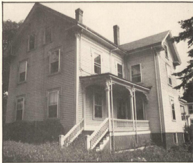
The Homestead House is defined by its shape, rather than by ornamental details. This house has decorative details borrowed from three styles: Greek Revival cornice returns, Italianate brackets, and Gothic Revival drip mouldings around the windows. Yet the house is essentially a simple Tri-Gabled Ell, typical of the Homestead Houses built in the 1870's.
