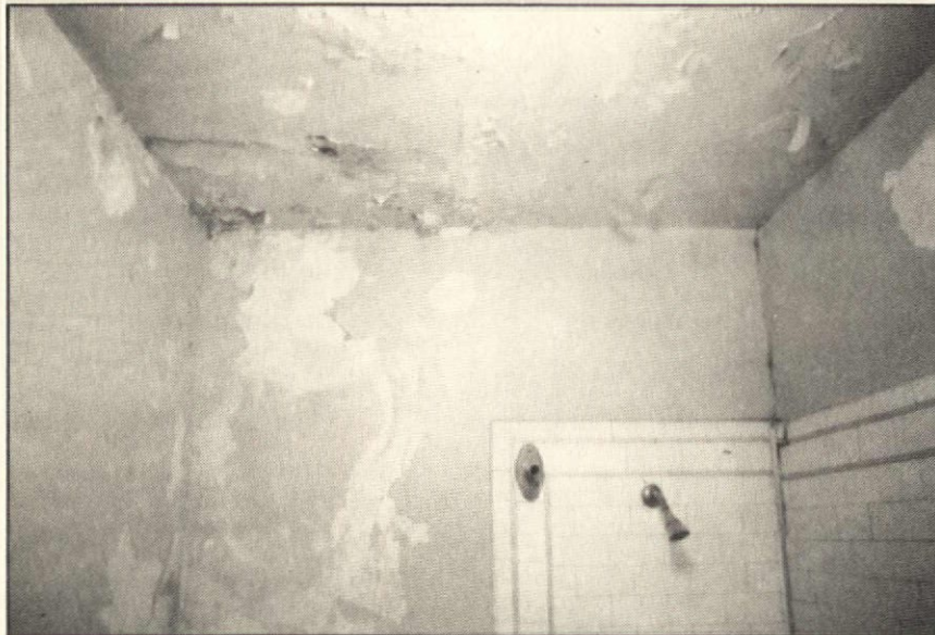
Above: When the walls and ceiling reach this condition, complete resurfacing is an answer. Below: This is the same room after the application of the Glid-Wall system.
