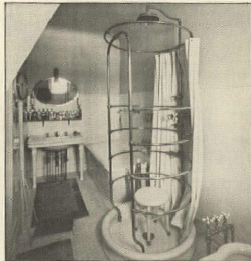
A 1909 bathroom complete with scale and an early shower unit.
