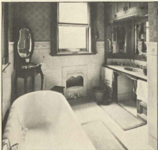
Notice the embossed tile and the built-in sink in this 1902 bath.
