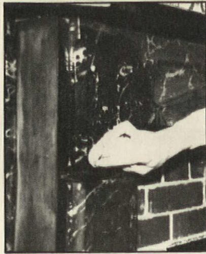
The essential step in removing the grime that obscured the original marbleizing (left) was nothing more complicated than washing with soap and water, followed by rubbing gently with fine steel wool (above). A coat of high-gloss varnish over the renewed finish (right) heightens the marble effect.
