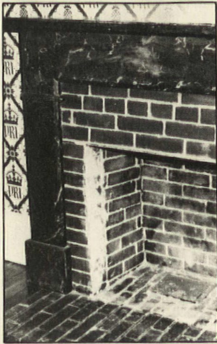
The essential step in removing the grime that obscured the original marbleizing (left) was nothing more complicated than washing with soap and water, followed by rubbing gently with fine steel wool (above). A coat of high-gloss varnish over the renewed finish (right) heightens the marble effect.
