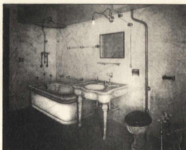
Until about 1900, bathrooms featured all the plumbing fixtures on one wall.
