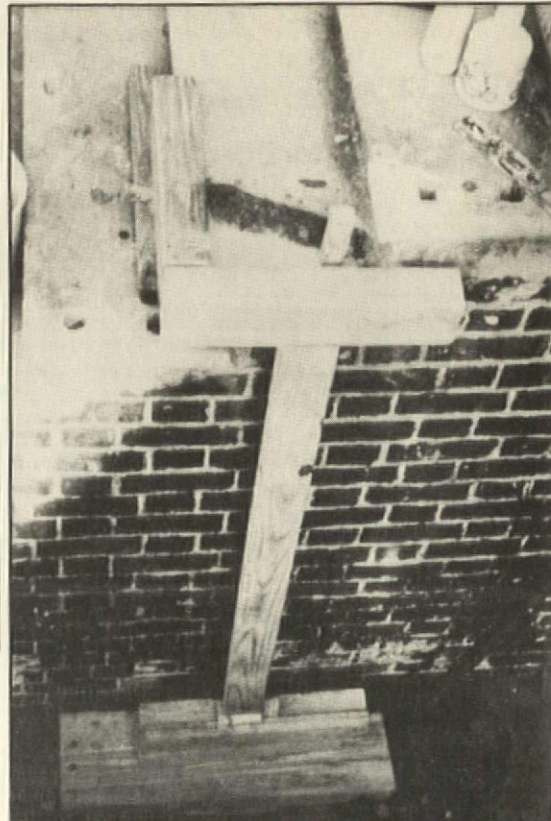
The finish coat of mortar is troweled into the wood forms, which are tamped into place on the step. Note the propping of forms, right. The block of wood near the edge is merely a spacer for a baluster that will be re-inserted later.
