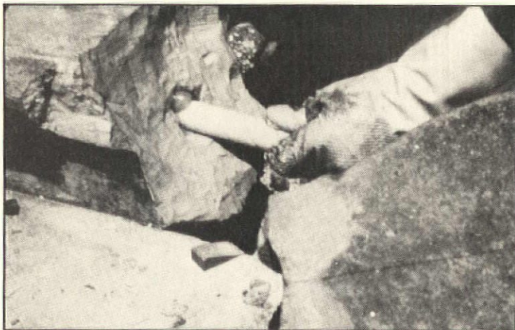
Matching holes are drilled in the step and its broken-off return. Then, a threaded steel or Teflon rod is used like a dowel to reinforce the connection. Epoxy acts as the adhesive for both the rod and the masonry bond.
