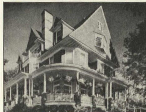
This view of the Rittenhouse Inn in Bayfield, Wisconsin, could only be made with a very-wide-angle lens due to constricted surroundings.
