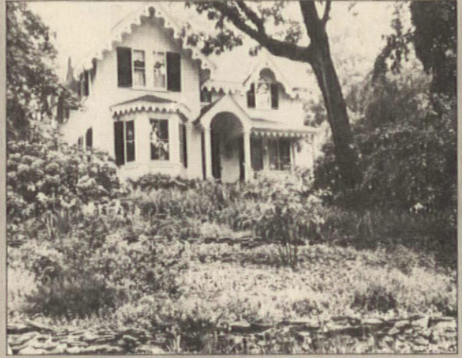
station. Above right is a recent photo of the house. The station is gone and a lot of trees have been cleared. Work remains to be done, but the house is definitely headed back to its original harmony with the landscape.
