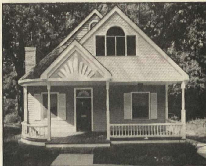
... involved, among other things, rebuilding the roof with a different pitch, and putting a completely new facade and porch on the house, all in an attempt to convert it into a "Victorian style gingerbread house." An honest Bungalow was remuddled into a caricature.
