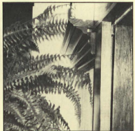
This side view of the new plate rail shows how the moldings were assembled.
