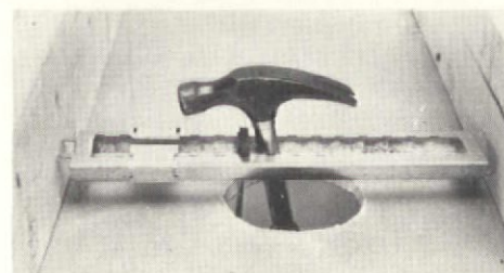
The 'Fan-Fast' support is installed with the aid of a hammer through a ceiling opening.
