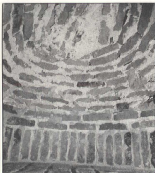
A pie's-eye view: This is the inside of the completed brick bake oven.
