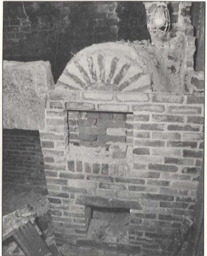
Above: After the mortar cured, the timber cribbing was removed; the lintel now is in place, spanning the firebox jambs. (Note the second lintel over the ash pit.) A soldier course of bricks lays out the floor plan for the bake oven.
