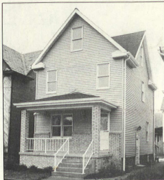
A TYPICAL REMUDDLING: small aluminum windows replace well-proportioned wooden ones, aluminum siding covers original clapboards, asphalt shingles supersede slate, wrought iron and fake brick take the place of the original porch. (photos courtesy of The Butler Eagle)
