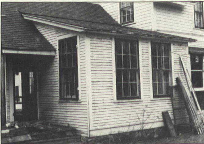
The Crosses kept the framed-in sunroom, but installed period windows and a new roof to make the room look like it belonged to the house.
