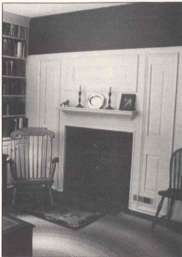
Nancy used two pine doors to make this fireplace surround. The left panel opens for storage.
