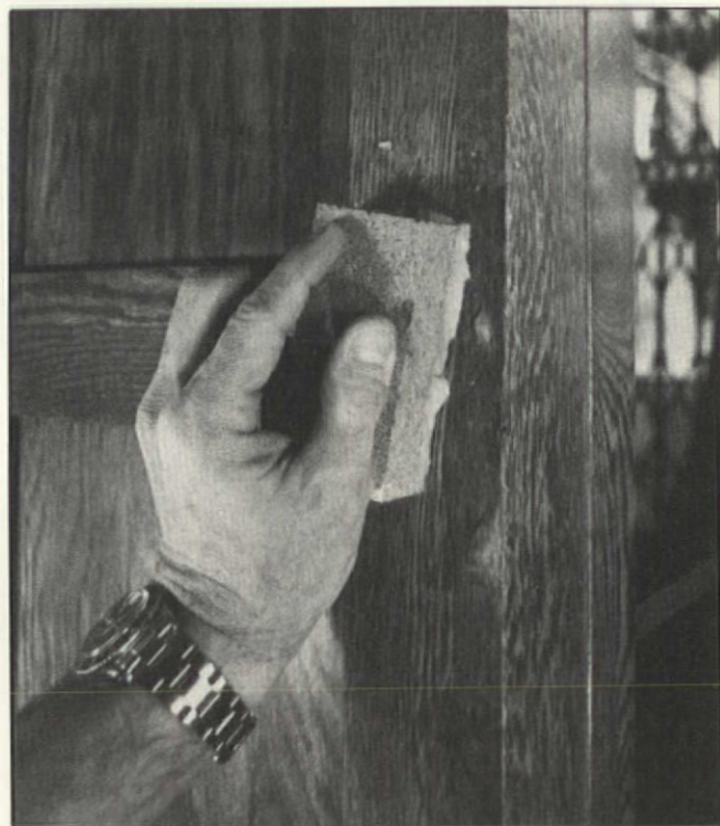
A thick cork block makes an excellent applicator for wood filler. It forces the filler deep into open pores and doesn't pull it out on the backstroke.
