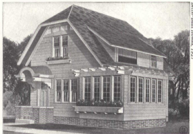
What makes one of the rooms under the dormer a sleeping porch, and the other a mere bedroom, is the unglazed window which is covered by only an awning.
