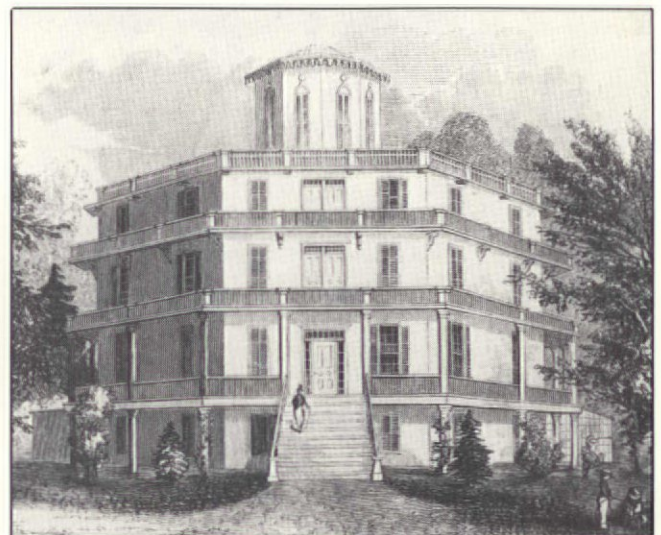
Fowler was no architect, but he was obviously fearless about following his own advice -- he designed and built this gravel-wall house for his family in Fishkill, New York. Alas, the 60-room residence, completed in 1853, no longer exists.
