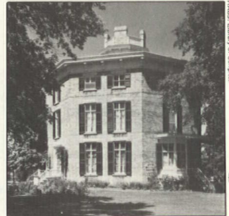
The John Richards House was built in Watertown, Wisconsin, in 1854. The largest octagon in the Midwest, it has 32 rooms and a central spiral staircase. (Note the octagonal cupola.)
