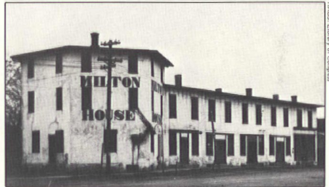
Orson Squire Fowler's model for the use of concrete walls in a polygonal structure was the Joseph Goodrich House, built in Milton, Wisconsin, in 1844.
