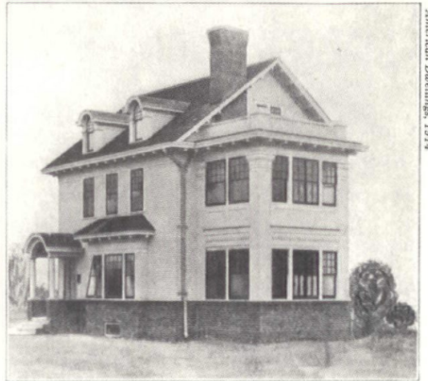
This neo-Federal has a typical sun room / sleeping porch wing that's "all sashed in, in case it gets too cool or starts to rain."
