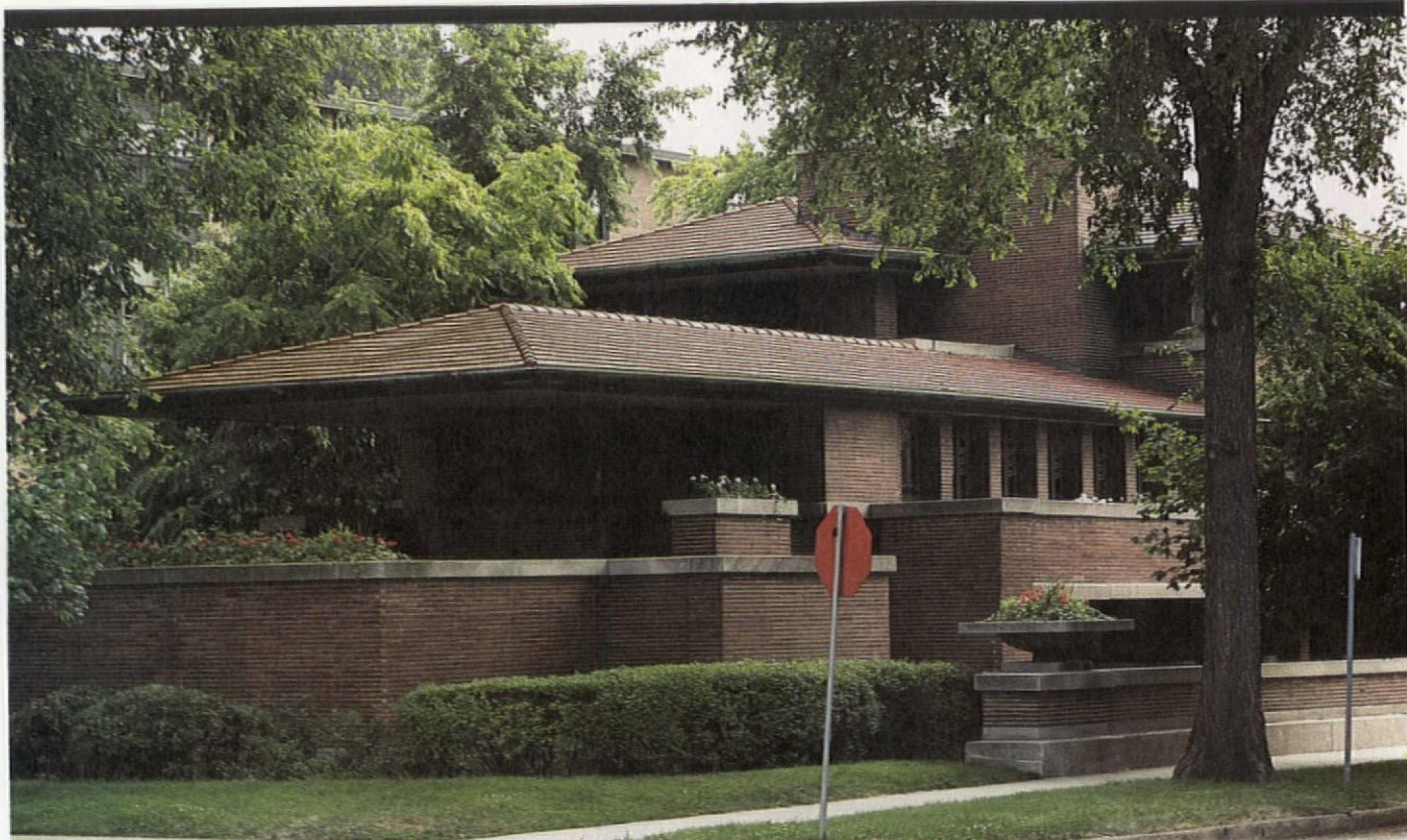
Frank Lloyd Wright's Robie House in Chicago still has its original 1909 Ludowici roof.
