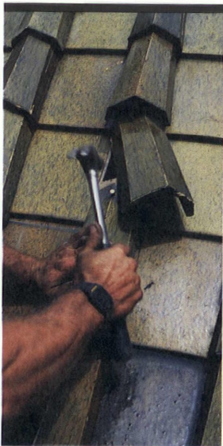
Resecuring a loose tile.
