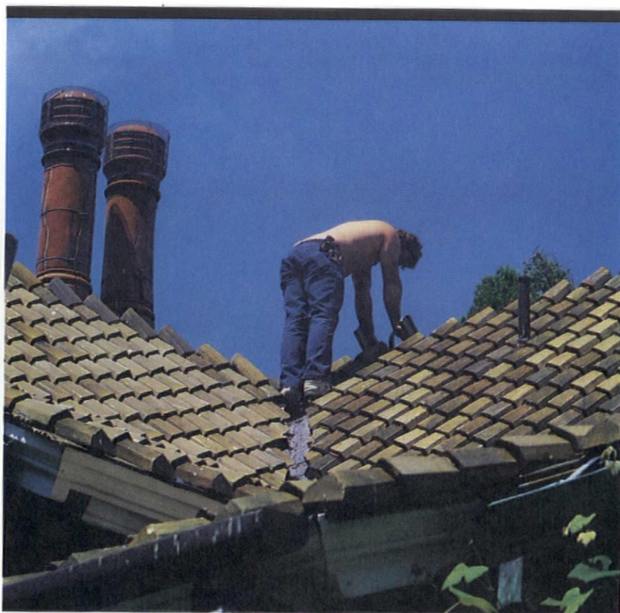
Greek pan tile is a variant of the Roman tile described on p. 23.
