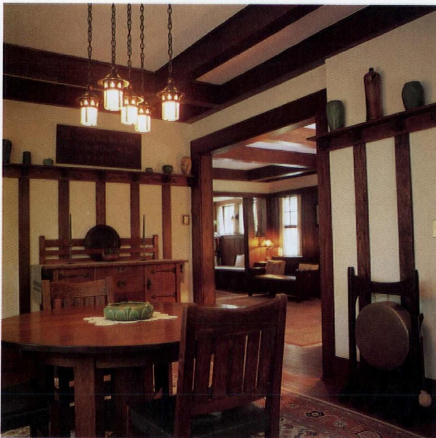
Ray rebuilt the plate rail in the dining room, above, based on unstained marks in the stripped woodwork.
