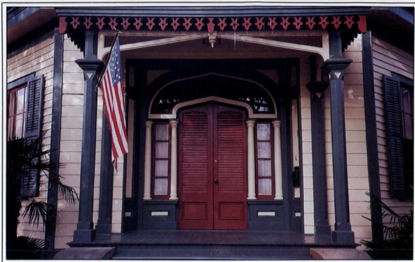
Gothic Revival is a style of details: In this doorway alone is an impressive Tudor arch, diamond-paned transom and sidelights, square columns, and simulated Gothic arches — actually artfully placed corner brackets.
