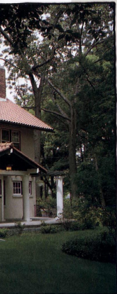
Craftsman House No. 104 today, left, and in a 1910 issue of The Craftsman, right. The plans called for a frame house with brick veneer and a slate roof. The Vaill family built their house in 1911 with ceramic cinderblocks and a Spanish-tile roof.
