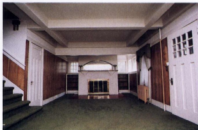
The living room before stripping began.
