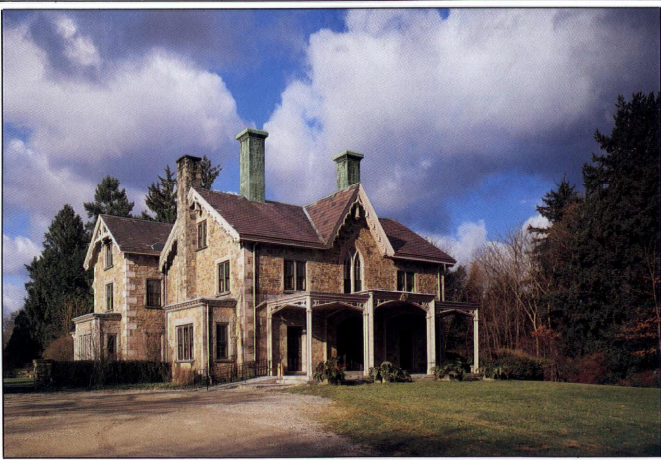
The Queset House in North Easton, Mass., above, was built 1854-55 "in the Andrew Jackson Downing style." Downing approved of prominent chimneys and porches on Gothic houses.
