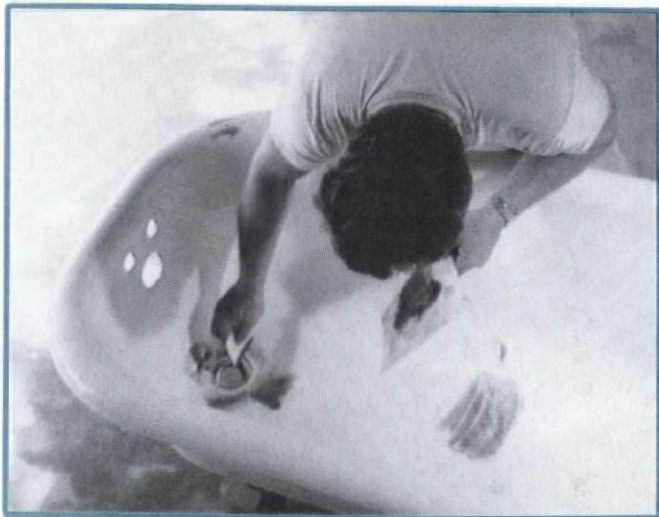
Nicks and scratches are filled with a fiber filler. This task requires skill, especially around the drain opening.
