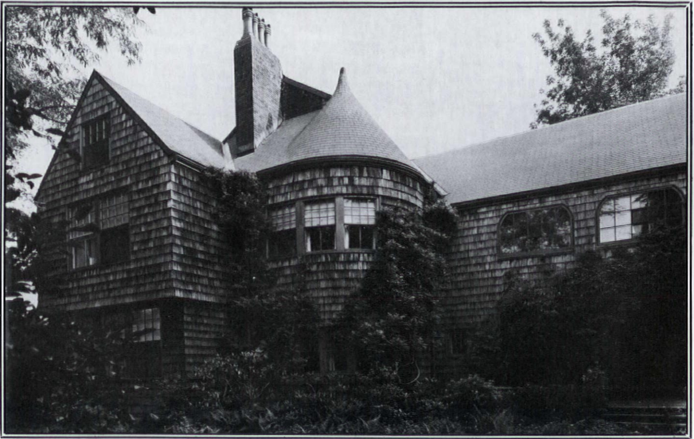
Shingle-style pioneer Henry Hobson Richardson designed this Cambridge, Massachusetts, home for Mrs. M.F. Stoughton in 1882. The shingled wrapping unites all the structure's elements into one smooth whole.
