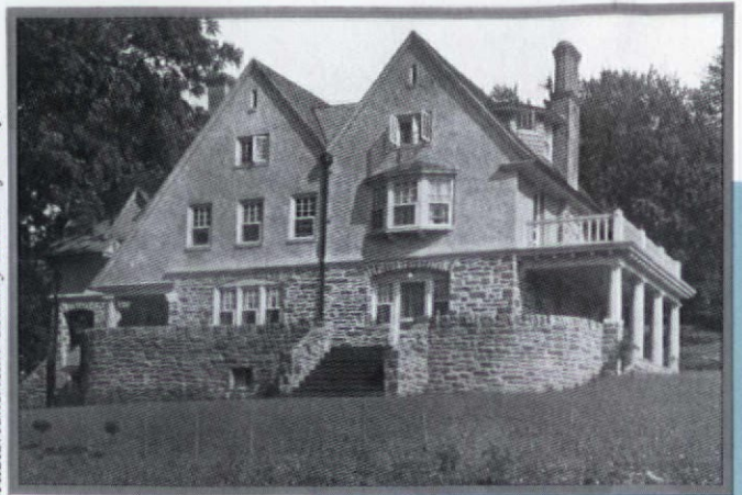
An oriel window at the rear brings light into an upstairs bedroom in this stone-and-stucco English Country house; Philadelphia, c. 1910.
