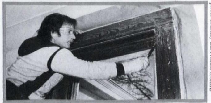
Stripping with chemicals requires protection for both window and worker.
