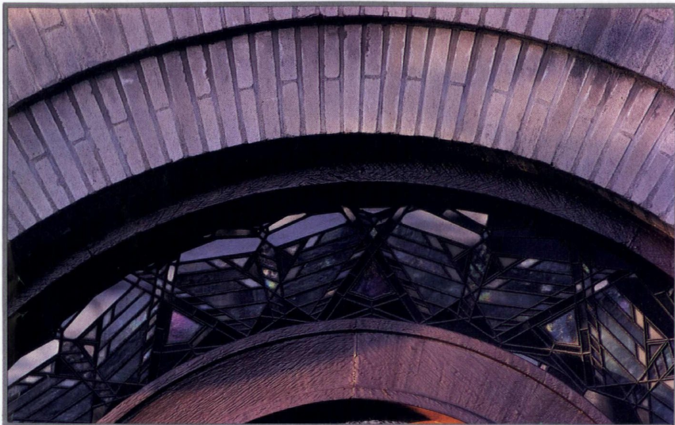
Exterior use of zinc "colonial came" on the Dana House, Springfield, Illinois; Frank Lloyd Wright, 1902.
