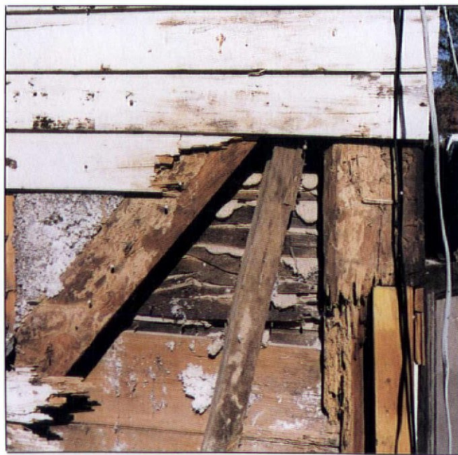
A close-up of the original siplap and lathing chinked with Georgia clay and pig hair.
