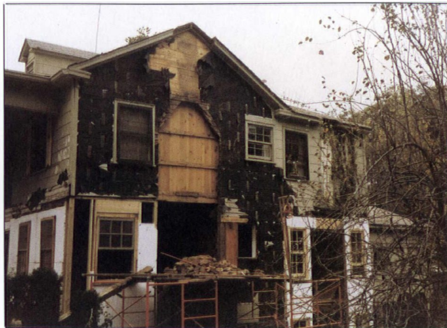
These gaping spaces were left when we tore out the dining-room and parlor chimneys and had them rebuilt using the original bricks.
