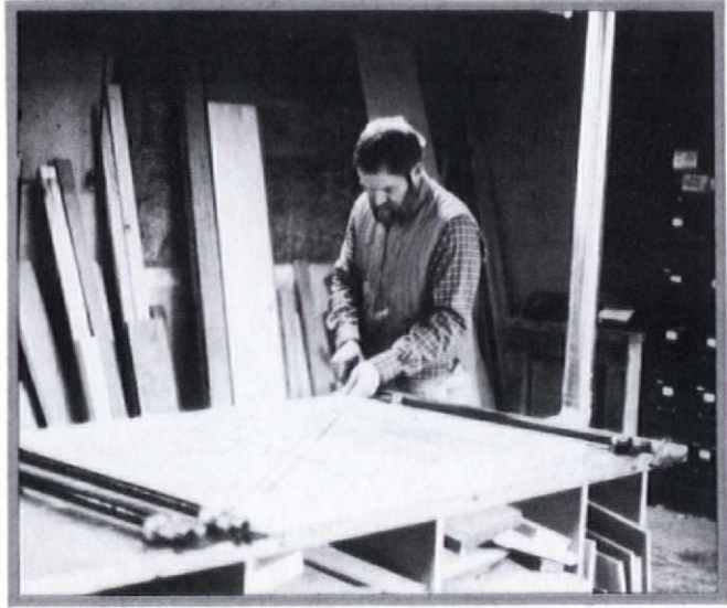
Fig. 4: Measuring the Diagonals
