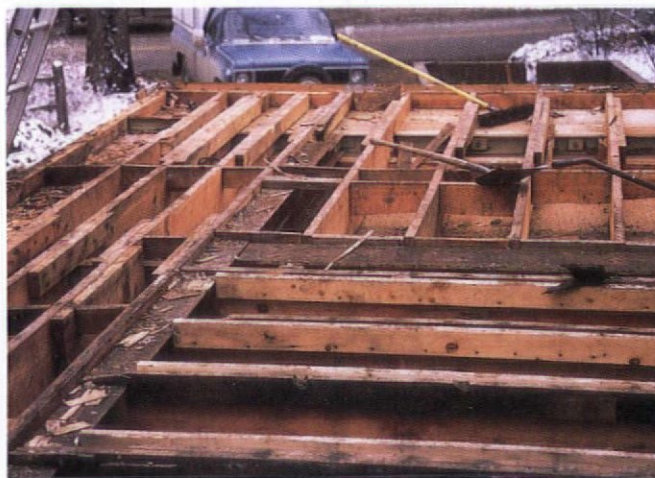
Mr. Wright's original framing along with the new framing is visible in this view of the lower roof over the carport (see Steel Framing Plan, far left).
