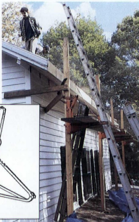
Ladder jacks (inset) will support scaffolding when used in pairs. Pump jacks (below) ride on 4x4 columns braced to the building.
