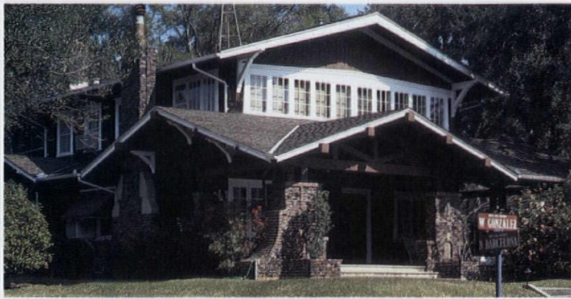
Left: Respect for natural materials is evident in the dark wooden walls and stone masonry of this substantial Pensacola, Florida, bungalow. Deep eaves shade an astonishing number of windows. Below: The porte-cochere at the Blacker House in Pasadena, California, built by Greene & Greene in 1907-09.
