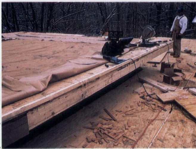
The membrane roof was on, above, but we went back when weather permitted to level and repair the fascia (see detail, page 44).
