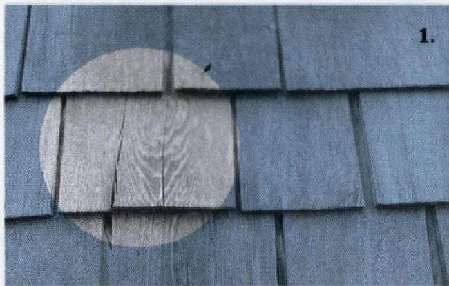
This shingle is suffering from two kinds of defects: a wind check on the left, and a weather check on the right.
