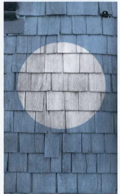
The bulk of these shingles are wide and flat-grained, and now plagued by weather checks.
