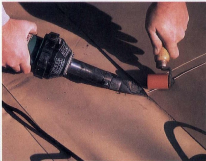
Mike Mason makes a field seam using a roller and Duralast's seam sealer which fuses the material with heat.
