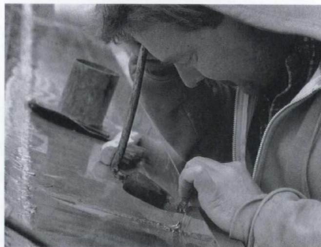
Soldering seams in a built-in copper gutter.
