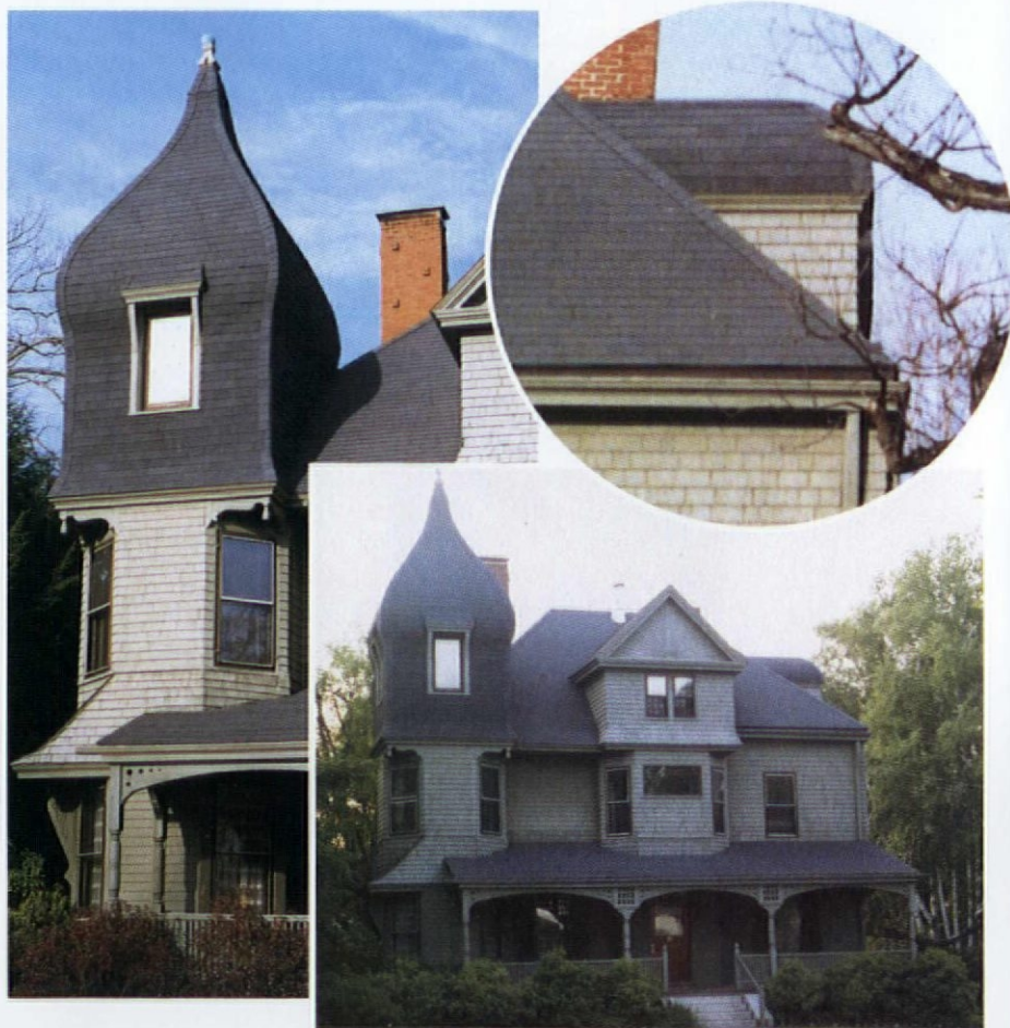
The shingles and siding of the tower (left detail) of the Alfreds' 1887 Queen Anne (right) may have matched that of the dormer (right detail).
