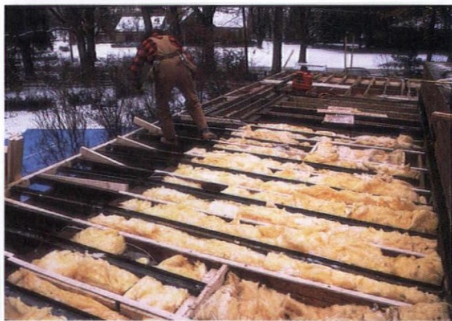
Four-inch steel channels are added to existing wood joists for support to the roof.
