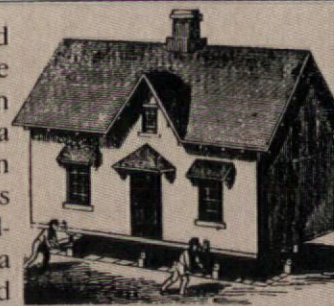
Raising with screw jacks, c. 1880
