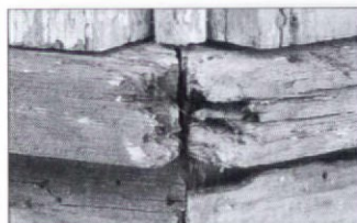
This rotted - and irreplaceable - woodwork...
