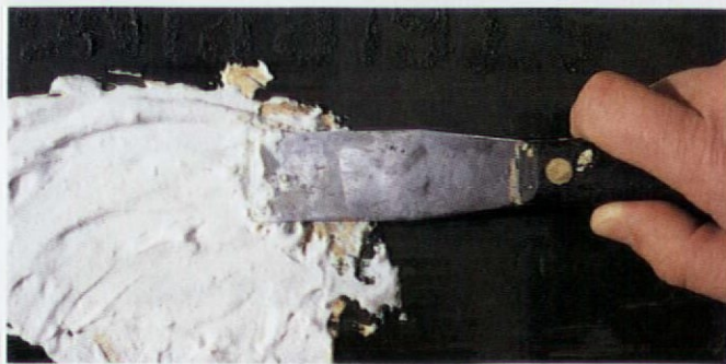
Caustic-based strippers are thickened into pastes when they are formulated for use on site. These strippers are applied by hand for most projects but may be sprayed on in commercial work.
