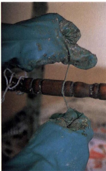
Strong twine helps remove softened paint sludge from baluster or furniture turnings. Chemical-resistant gloves should be worn.
