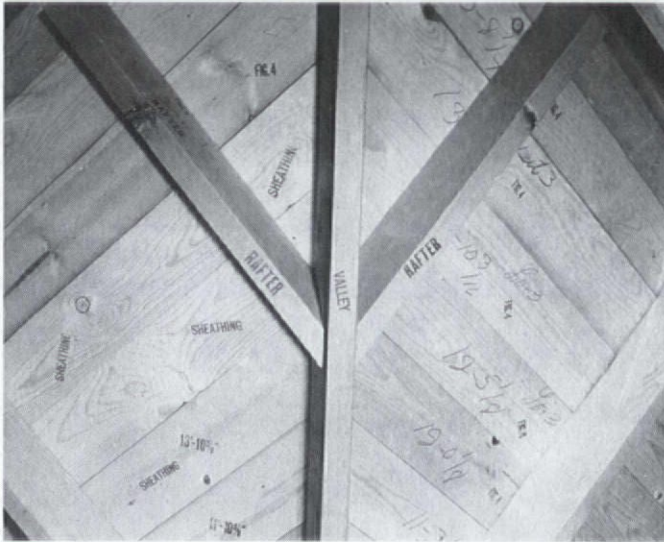
If you're curious about whether you own a ready-cut house, look in the attic space — the names of the parts were often clearly marked.
