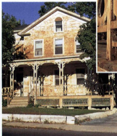
The caustic strippers are popular for exterior stripping, but they may also produce "fuzzy grain" on certain woods.
