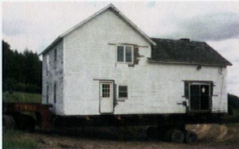
"Going three points": two dollies (at rear) and the tractor's fifth wheel.
