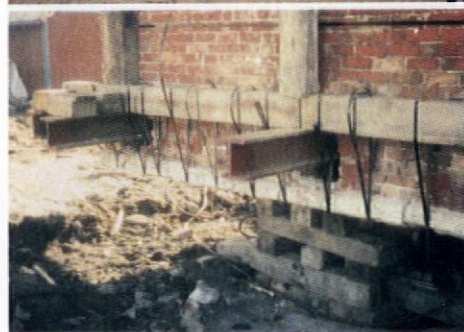
Top: preparing a cut house. Above: steel banding used for masonry.
