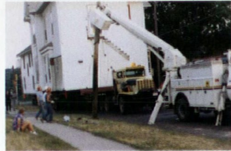
Utility lines — and even poles — are common, expensive obstacles.
