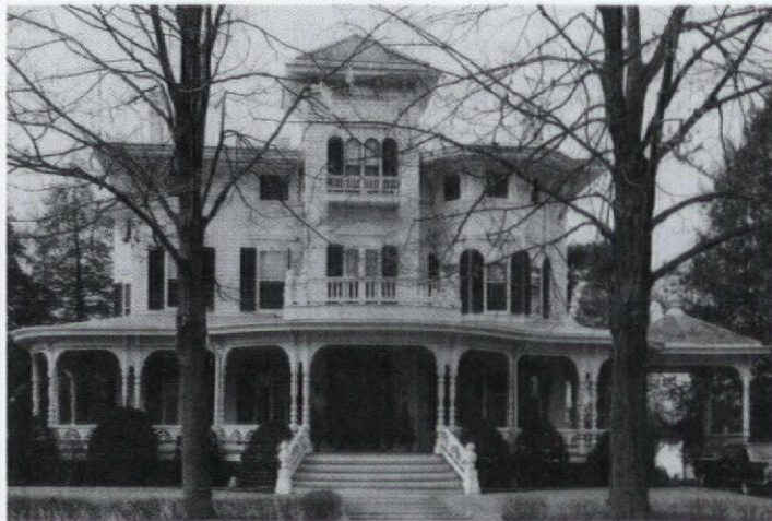
Shipbuilding is the decorative key to this handsome Italianate and its wrap-around porch.
