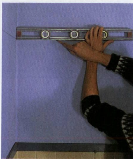
Leveling lines comes into play when laying out projects such as cabinetry, tilework, or even wallpaper.
