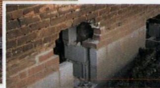
A new foundation and holes left by steel.
