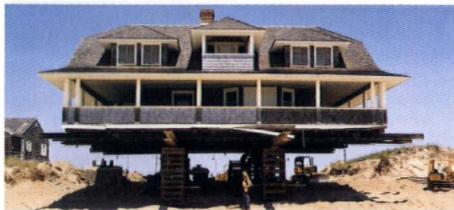
Supported entirely by cribbing and steel, this seaside house awaits its new foundation.
