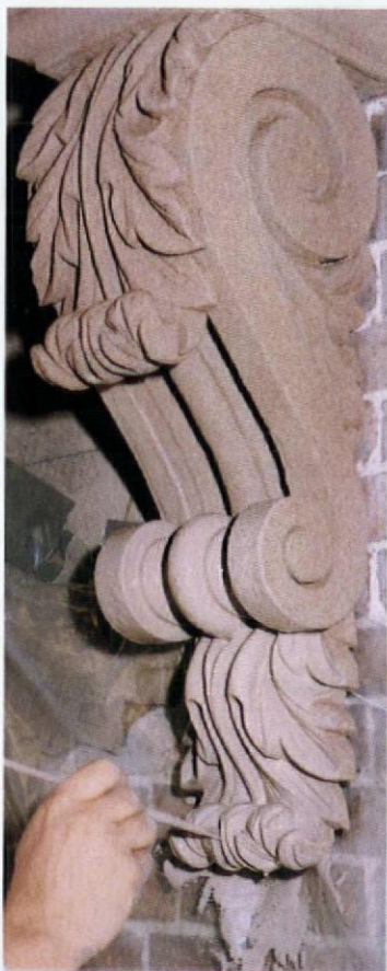
While the already sanded upper scroll dries, the lower leaves of this console get a thick touch-up coat of oil-based paint.
