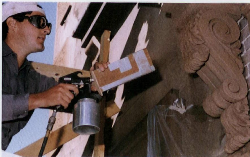
Sand is blown onto the fresh wet paint of this console with a V-trough and compressed air. A sandblast cup at the end of the hose provided just the right control of air, but sand was still supplied from the trough.
