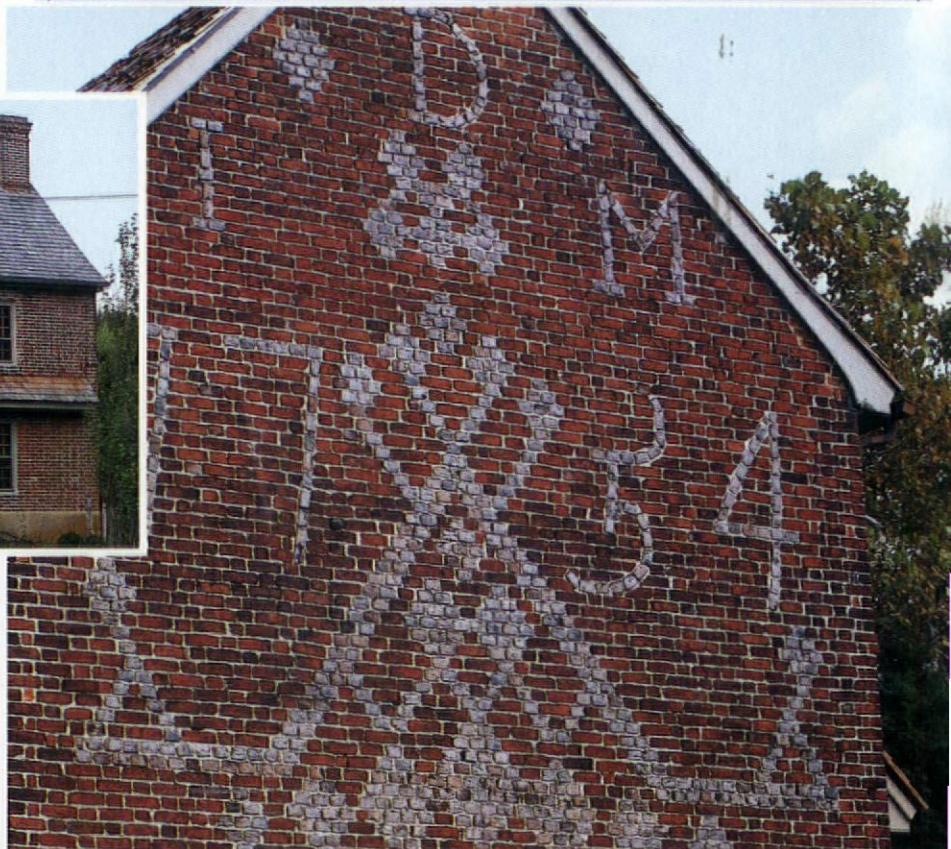
Salem County brick patterns, top to bottom: dramatic zigzag (William Hancock House); diamond or diaper (Abel Nicholson House); Flemish bond (Abel Nicholson House). Above, the typical I-House form of the John Dickinson house and, at right, its highly expressive end wall.
