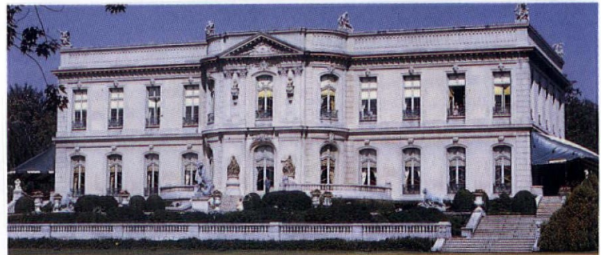
Top: An Italian/Mediterranean interpretation of the Beaux Arts in Palm Beach, Florida (Flagler Mansion, 1901). Middle left: The mansard roof is a hallmark of French-style Beaux Arts buildings, here in Washington, D.C. (Fabnestock House, 1909). Middle right: White marble columns, cherubim, swag, cartouche, and urns are typical of the sumptuous doorway adornment (DeLamar Mansion). Above: In the best Academic Eclectic tradition, the garden facade of Edwin Berwind's Newport summer home interprets rather than copies the small chateau on which it is modeled ( The Elms , 1901).
