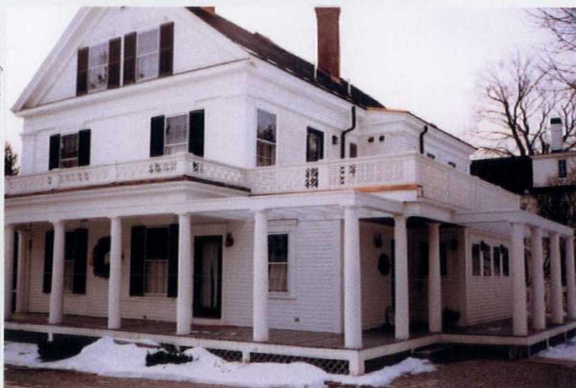
The new railing (center and right) on the roof of the rear addition visually matches the original railing (left) on the side porch roof.
