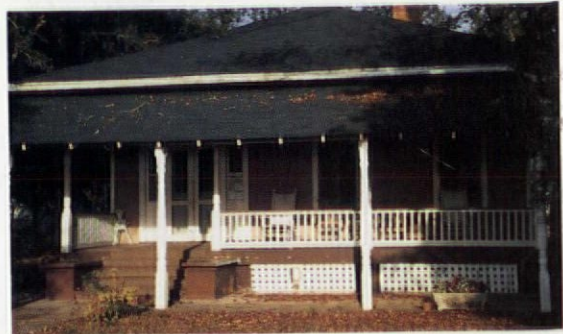
A rain porch is an architectural accessory that keeps driving coastal rain off a variety of building types, such as this c. 1900 Victorian house.
