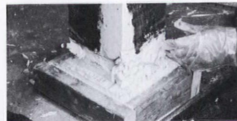
...were completely sawed off and replaced with...
