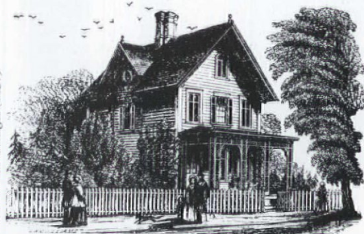
The central chimney (for efficiency) and side gable (for staircase headway) made this simple Vaux cottage a highly buildable design.
