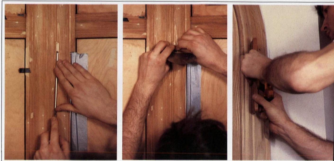
Shaping steps (left to right): paring a dutchman flush with the moulding using a cranked-neck chisel; fine surfacing with curved
