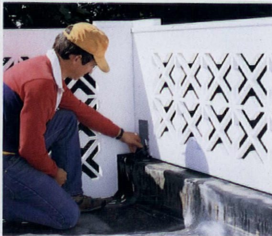
Custom-fabricated steel brackets (left) support the railing and tie it to the roof structure. The brackets were mounted over the already-laid, modified bitumen roofing, and then sealed with another layer of roofing (right).
