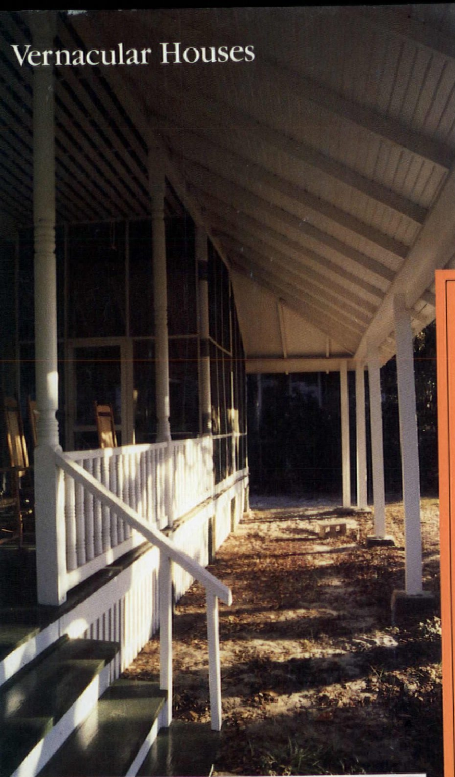
A rain porch is an architectural accessory that keeps driving coastal rain off a variety of building types, such as this c. 1900 Victorian house.
