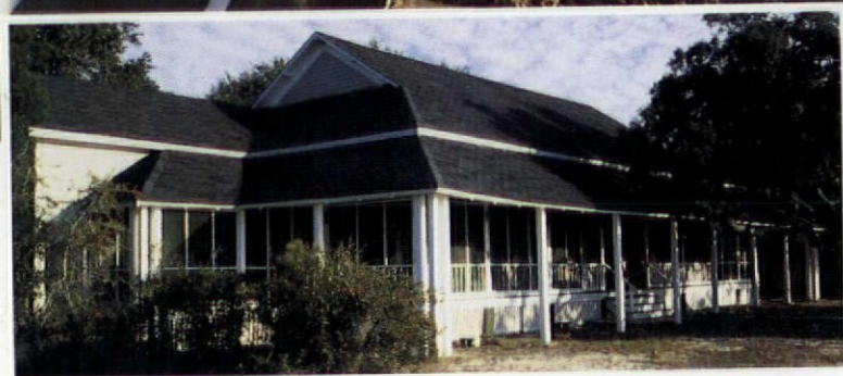
The extended roofline created by a rain porch can be seen on this 1895 Point Clear house (inset). Above: an interior view of that house's rain porch. Note the slatted porch ceiling on the galerie for ventilation.
