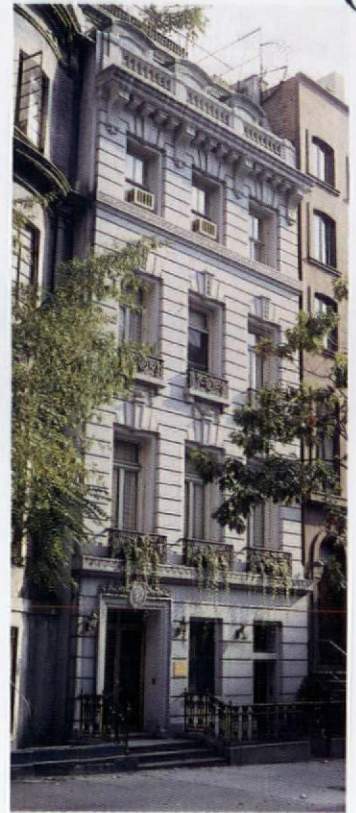
In this five-storey New York City townhouse, iron balconies, all-over rustication, and a full-width stone balustrade at attic level provide horizontal balance as well as elegant ornament.
