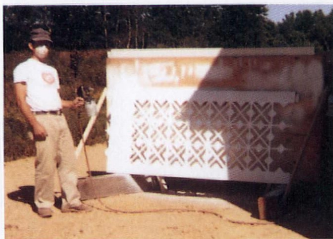
Painting one of the individual sections which incorporate a top and bottom rail and one post.
