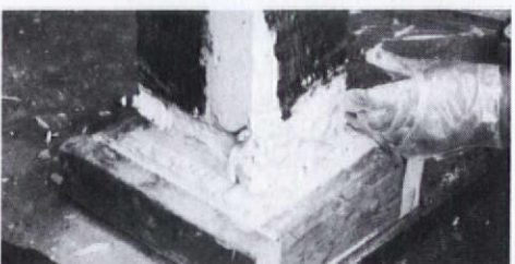
...were completely sawed off and replaced with...
