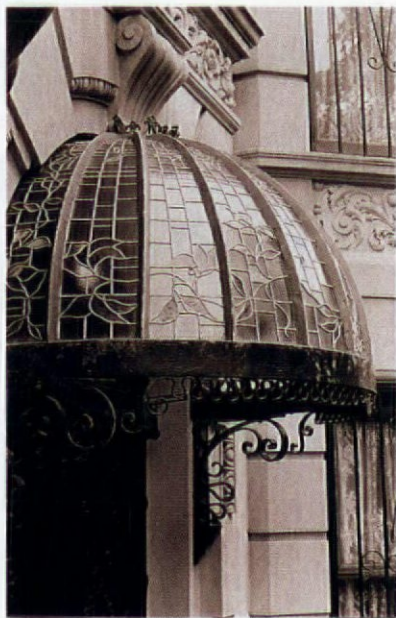
This delicate stained glass canopy, designed by Alpat Studios, creates an impressive entryway.
