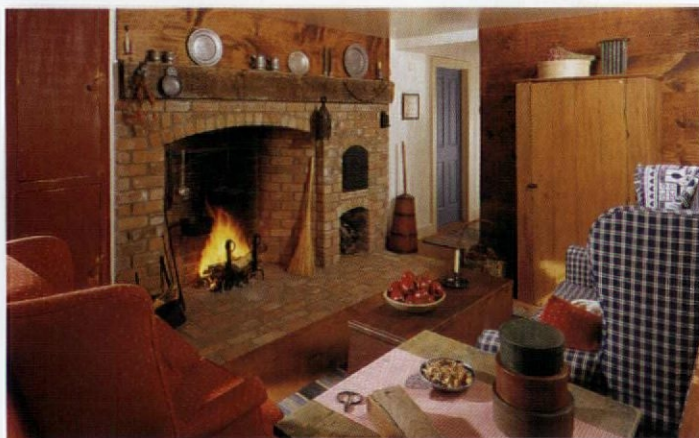
Note the wooden mantelshelf set above this early-18th-century fireplace.
