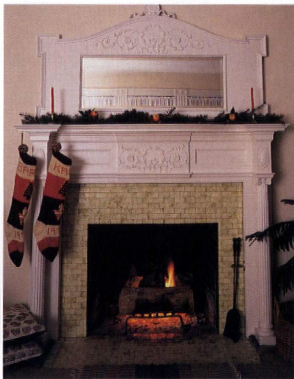
Final surface components, such as decorative tile surrounds and the mantelpiece itself, are applied to the leveled breast to complete the job.
