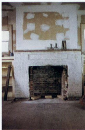
A "surgical" firebox demolition.
