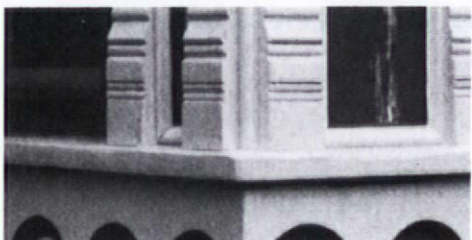
...sanded, nailed, stained or painted.
