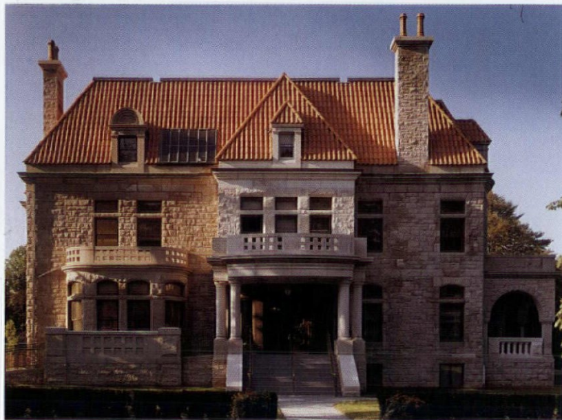
For the added portico on this 1887 house — home of the Preservation Society of Newport County, Rhode Island — matching materials were used, but the detailing — geometrical rather than round balusters — differentiates it from the original building.
