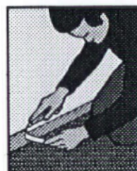
5. Trim mat at baseboard and window.
