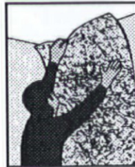
3. Apply fiberglass mat to wet surface.
