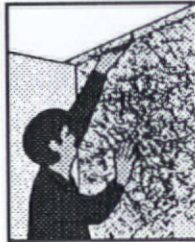
4. Trim excess mat where wall meets ceiling.
