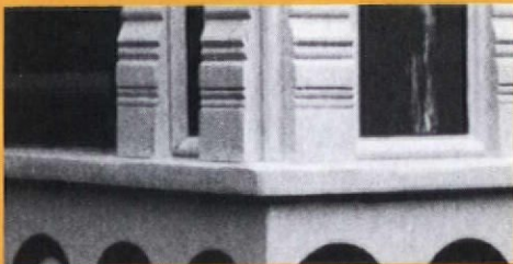
...sanded, nailed, stained or painted.
