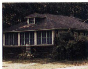
A filled-in porch turns a classic bungalow into just a box.
