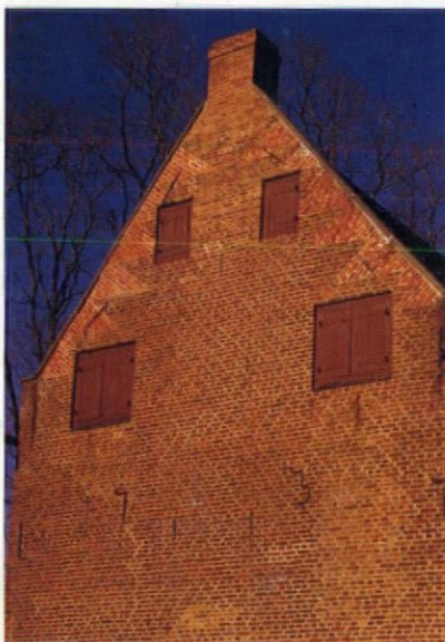
Mouse tothing — the defining feature of Dutch brick houses — can be seen on the parapet-gabled end of the Van Alen House in Kinderhook, New York.
