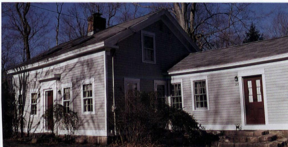
ABOVE: A reduced scale subordinates the proposed annex to this 18th-century Greek Revival house at Williams College. The connecting “hyphen” limits changes to the historic fabric. RIGHT: Setbacks have long been used to subordinate additions. Both main house and extension were built in the 1840s for the daughter of a pea farmer in Mount Carmel, Connecticut. The wing served as a buttery and contained an indoor well.
