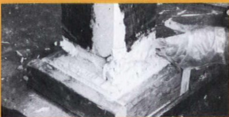
...were completely sawed off and replaced with...
