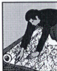
1. Cut fiberglass mat 2" longer than height.
