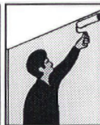
12. Apply 2nd coat of saturant (include seam)
