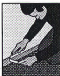
5. Trim mat at baseboard and window.
