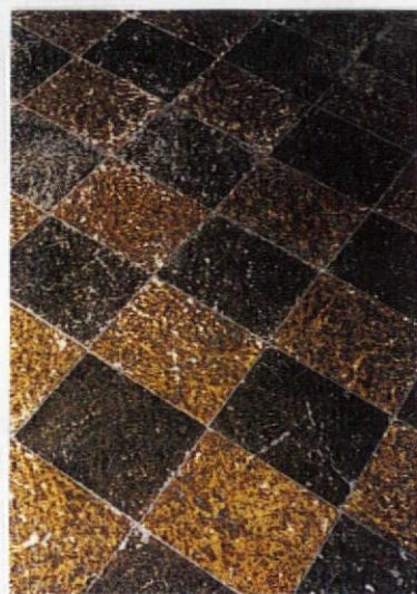
The Botticellis' floor looks like Zenitherm, a man-made product that resembles honed stone tile.
