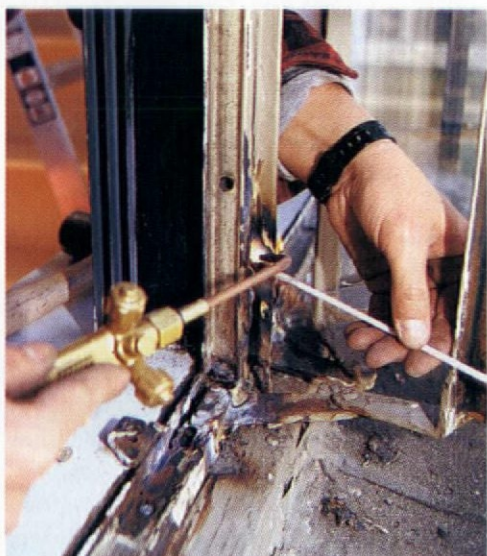
Make sure the metal frame is strong enough to anchor the hinge. Then weld it in place, taking care to position it properly.
