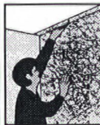
4. Trim excess mat where wall meets ceiling.
