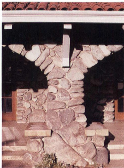
The distinctive river-stone masonry arch and picturesque pillar base figure in many western bungalows, but especially in the “grove houses” of the citrus-growing area around Claremont, California.
