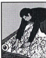
1. Cut fiberglass mat 2" longer than height.
